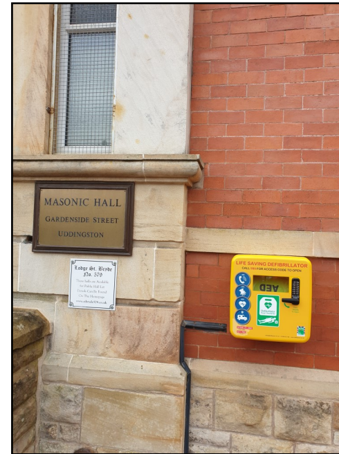
The unit mounted on the outside wall of our Hall.
