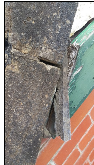
Left. Deterioration above the lounge window. Right. Top coping stones being removed above lounge window and re-bedded.
