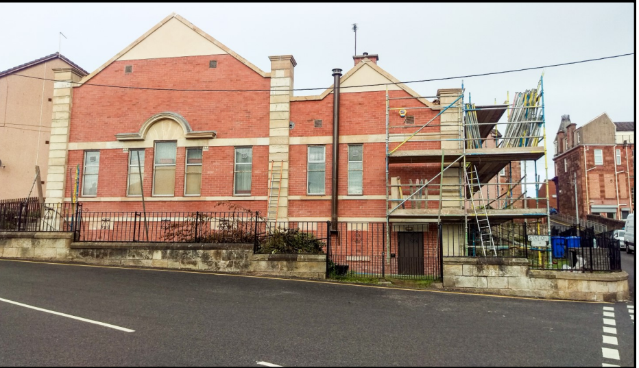
West Wall complete !
