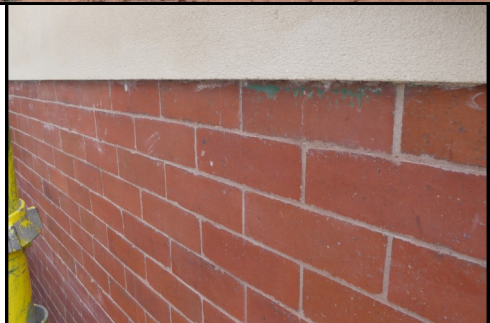
Re-pointed brickwork and sandstone cleaned on West Wall.
