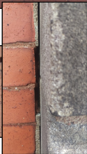
Re-pointed brickwork and sandstone cleaned on West Wall.
