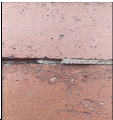
Examples of the deterioration found in the West Wall mortar.
