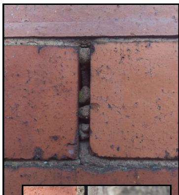
Examples of the deterioration found in the West Wall mortar.
